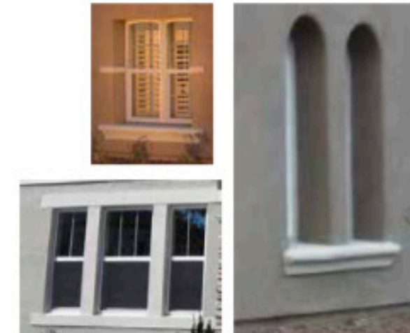
5. Window Header & Sill Detail
