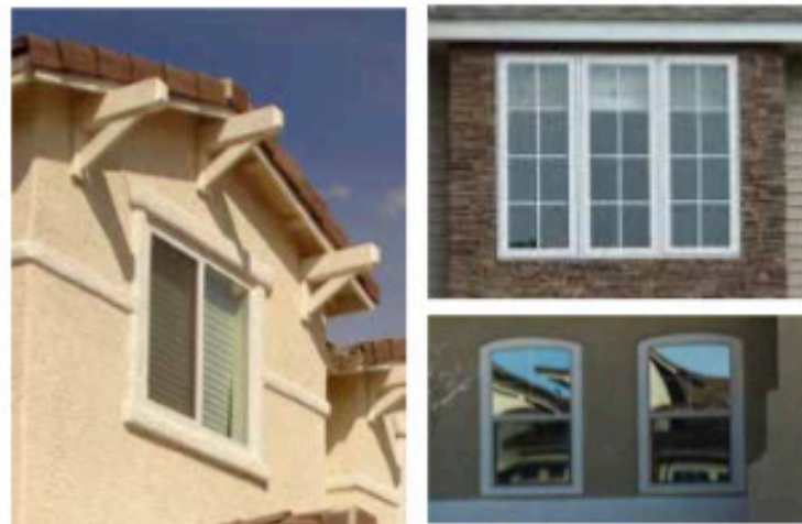
4. Window Casing Detail
