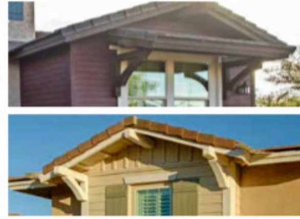
2. Gable End Window Detail with Corbels
