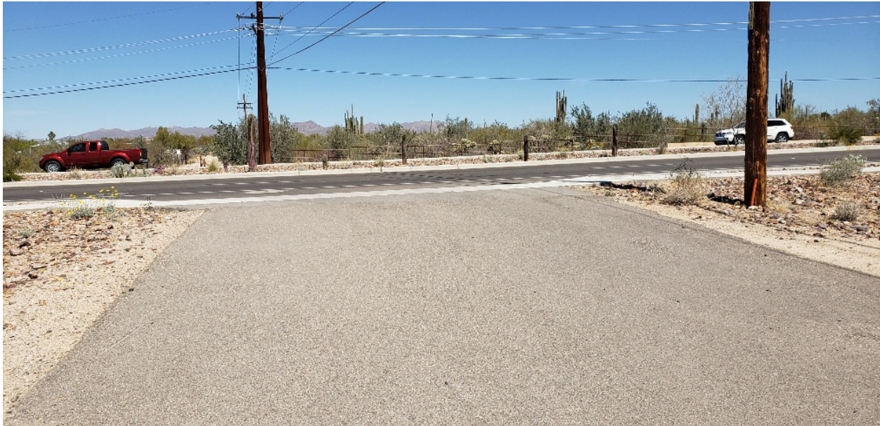
Looking North on Camino de Oeste Curb Cut toward Cortaro Farms Road
